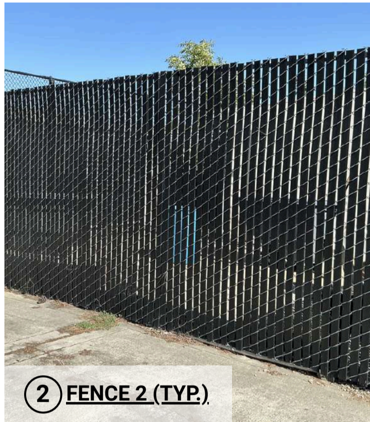
FENCE 2 (CHAINLINK) (PANELED) MAINTAIN EXISTING FINISH
