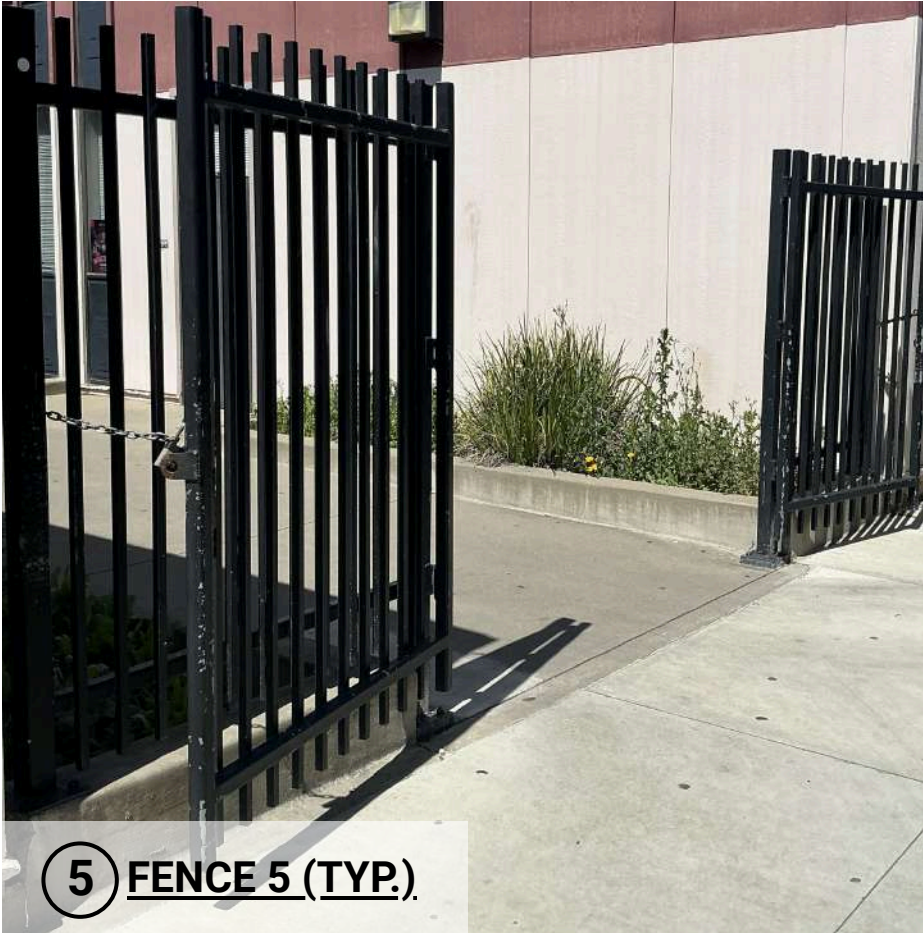
FENCE 5 (ORNAMENTAL STEEL) PAINT COLOR
