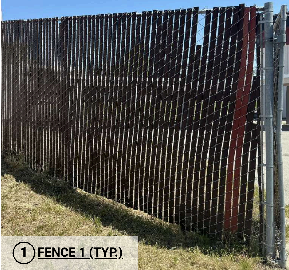
FENCE 1 (CHAINLINK) (PANELED) MAINTAIN EXISTING FINISH
