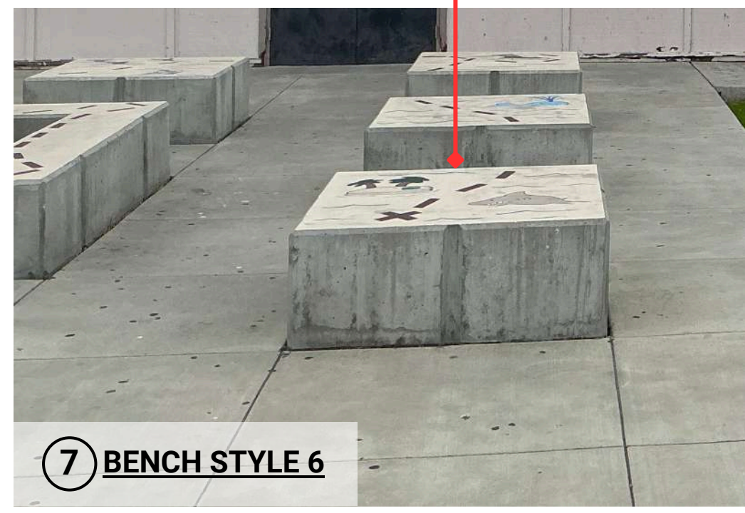
CONCRETE PLANTERS (TYP.) SANDBLAST & APPLY SEALER
