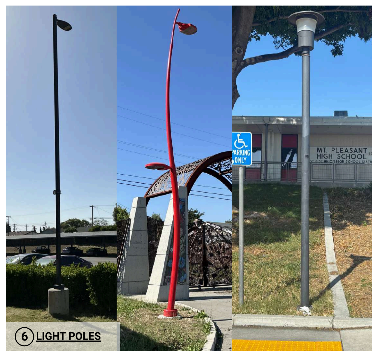
LIGHT POSTS (TYP.) MAINTAIN EXISTING FACTORY FINISH ON LIGHT POST & CONCRETE BASE
