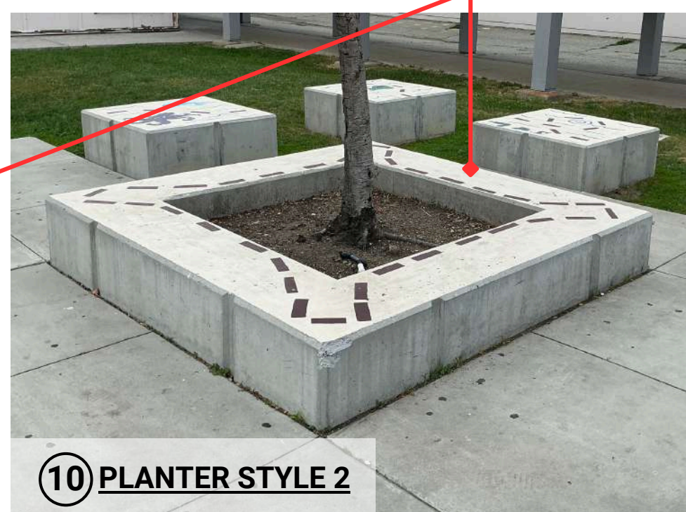
CONCRETE PLANTERS (TYP.) SANDBLAST & APPLY SEALER
