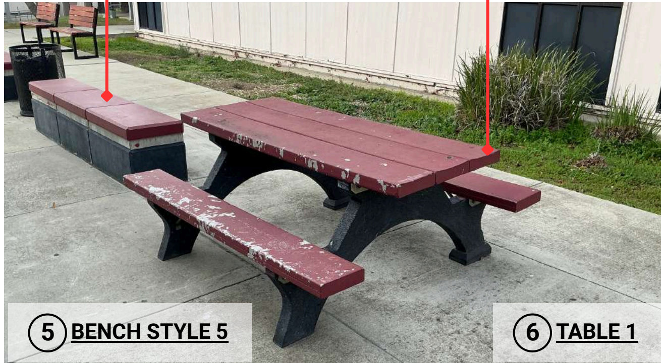
BENCH STYLE 5 (CONCRETE W/ PAINT) SANDBLAST & SEAL
