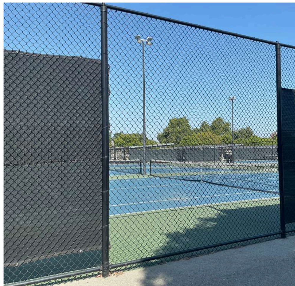
FENCE 3 (METAL) (CHAINLINK) (PAINTED) MAINTAIN EXISTING FINISH
