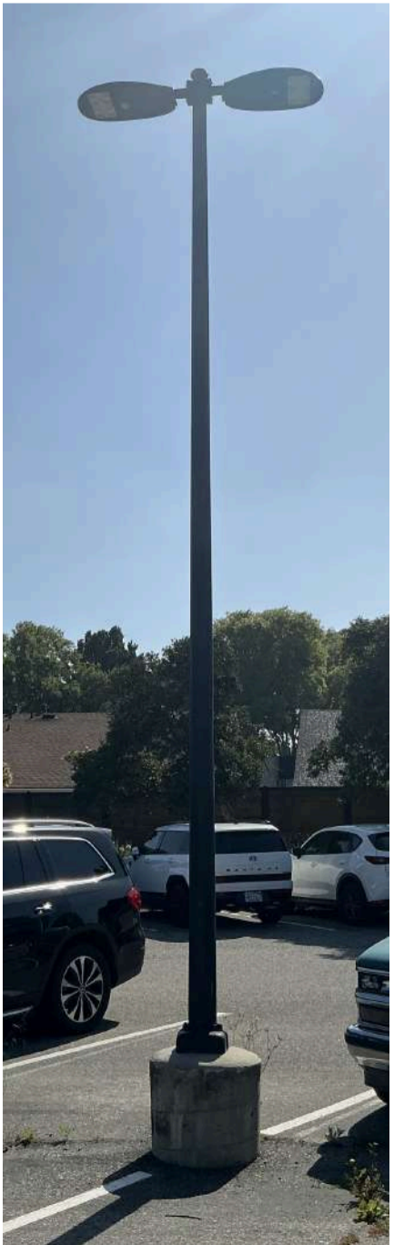
LIGHT POSTS (PAINTED) (TYP.) PAINT COLOR AND MAINTAIN EXISTING FINISH ON CONCRETE BASE
