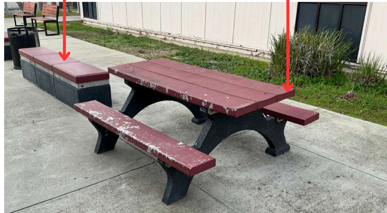
BENCH STYLE 3 (CONCRETE W/ PAINT) SANDBLAST
