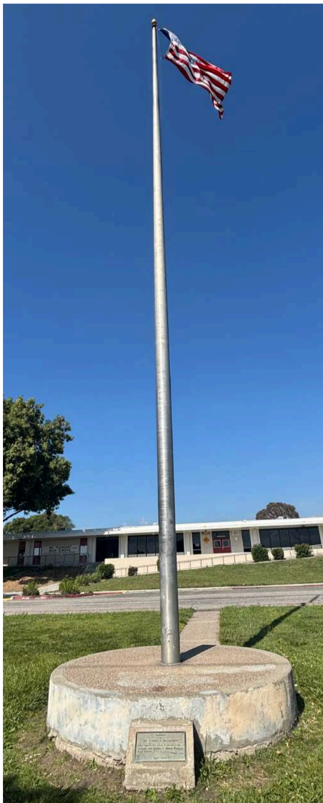
CONCRETE BASE SANDBLAST & RESTORE TO BAREFORM, PROTECT DEDICATION STONE
