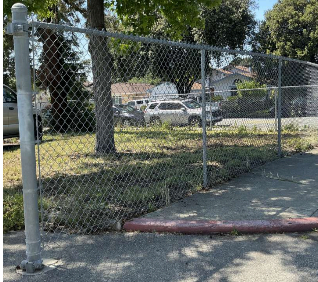
FENCE STYLE 2 (CHAINLINK) (UNPAINTED) MAINTAIN EXISTING FINISH
