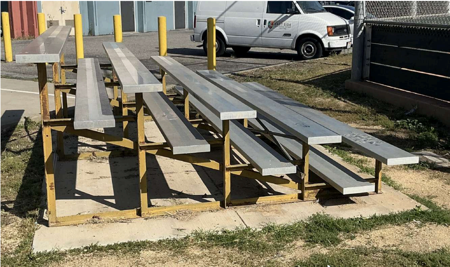
BLEACHERS WITH PAINTED BASE (METAL) (TYP.) PROTECT IN PLACE
