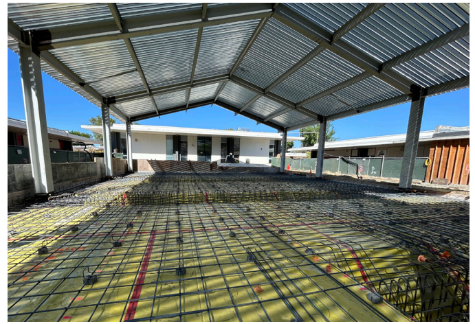
Construction Progress of Building 500
