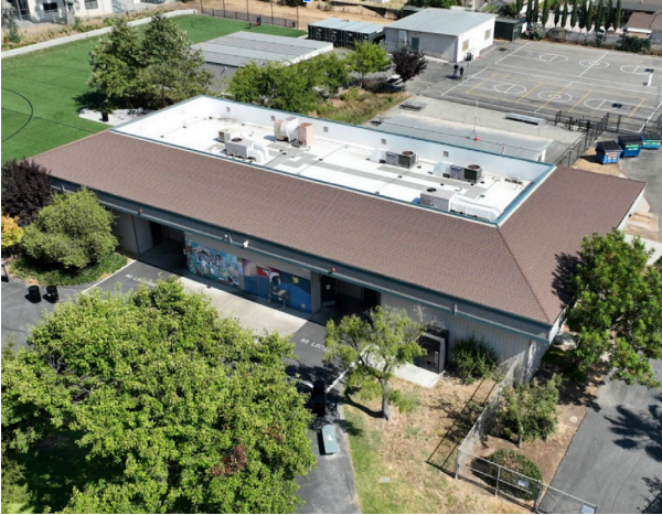
Building G Exterior
