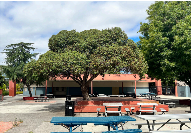
Pre-existing Building K
