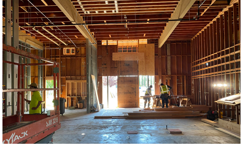
Construction Progress – Interior
