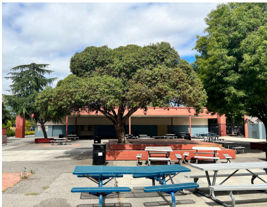
Existing Building K
