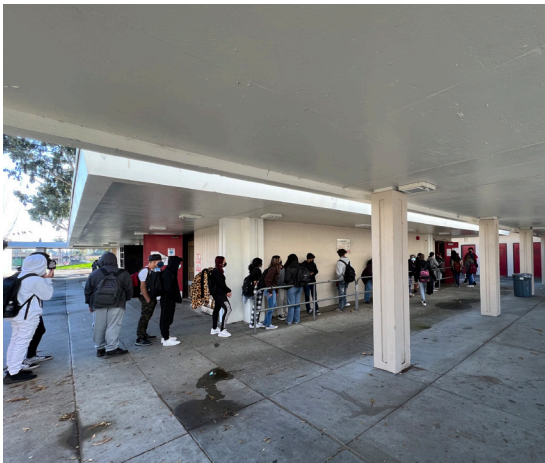
Existing Food Service Building
