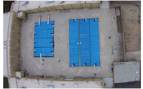
Aerial Before Photo of Mt. Pleasant
