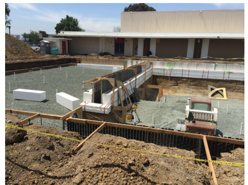
Mt. Pleasant Pool Construction: Island Dividing Shallow and Deep Pool
